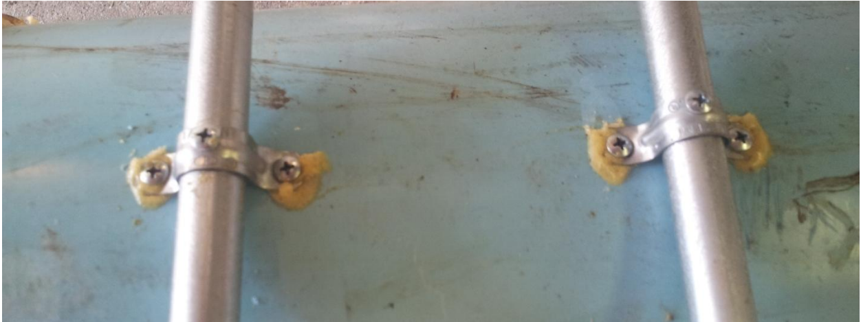
Figure 37– Conduit Held to Floating PVC
